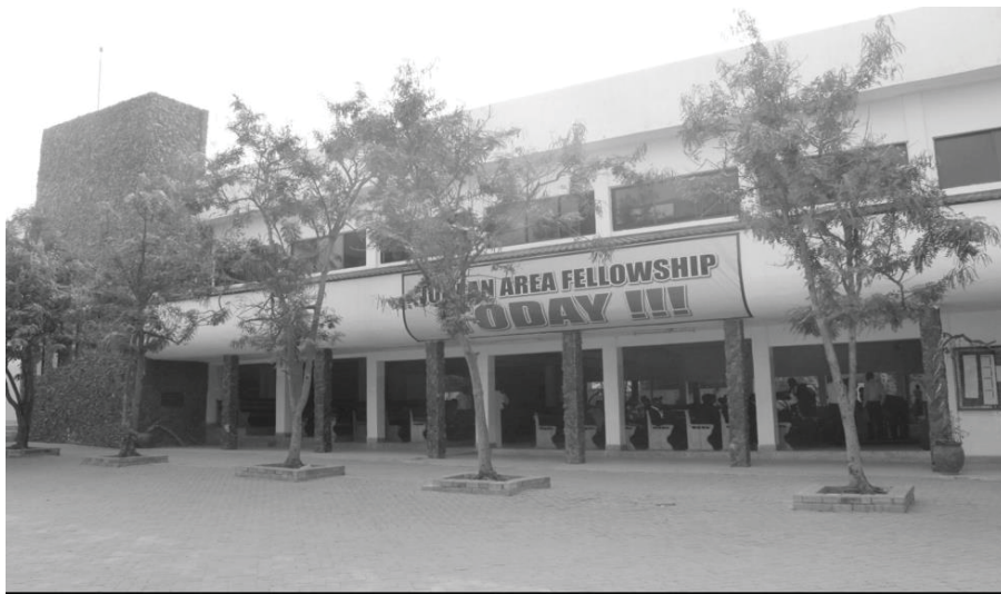
Photo 7: LCI Korle-Gonno Cathedral showing the open space open window architecture (Credit: Author).
